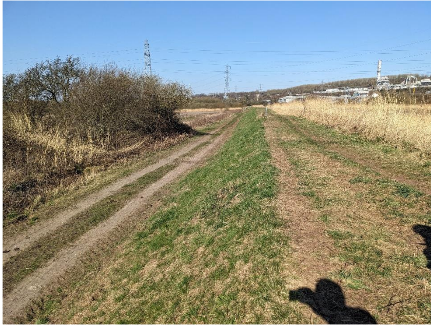
Landward Face Southern Reach
