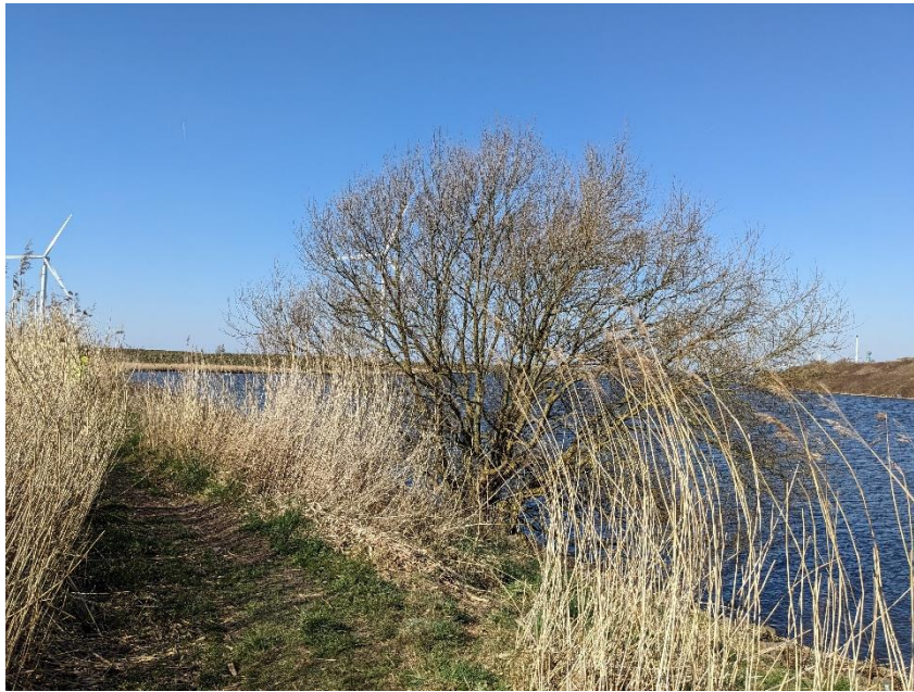
Exposed Face Centre of Embankment
