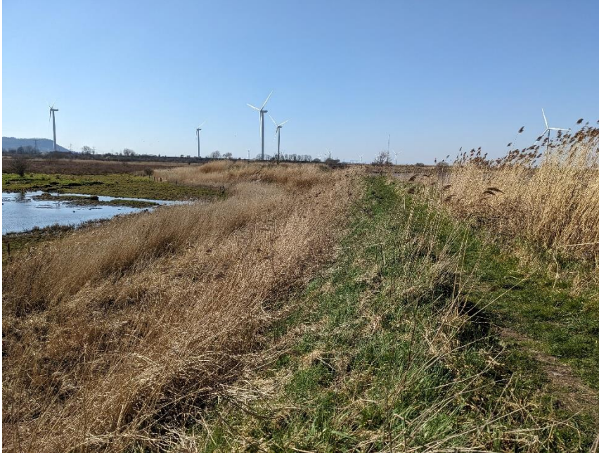
Landward Face Southern Reach
