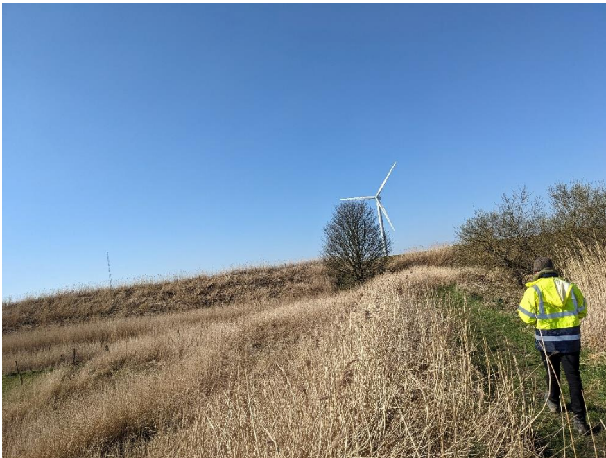
Landward face Northern Reach
