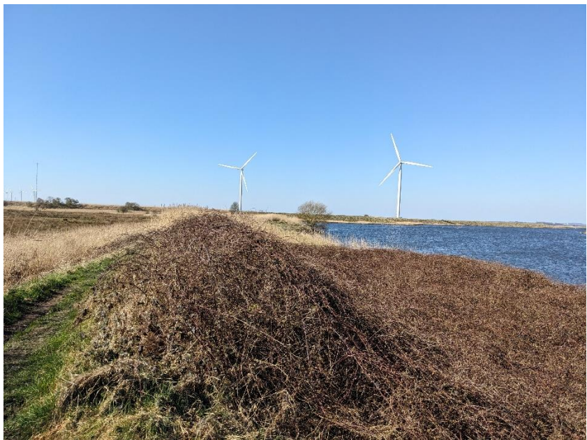
Exposed Face Northern Reach
