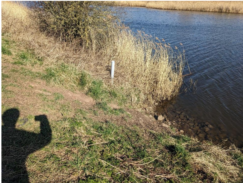
Exposed Face Centre of Embankment
